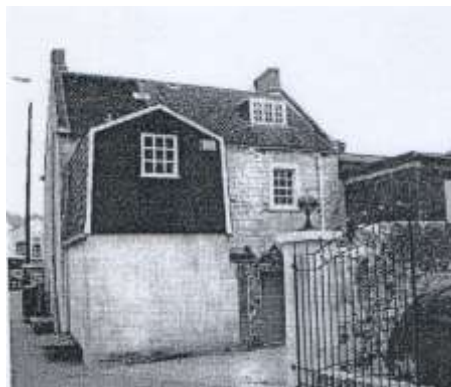
REAR VIEW SHOWING TWO-STOREY EXTENSION
